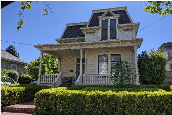
Figure 15. Residence on D Street that is outside the A Street Historic District.
